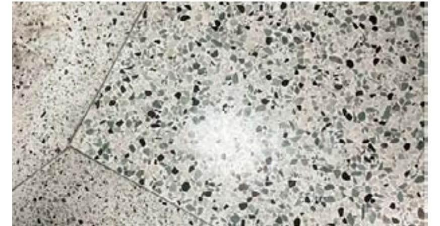
Existing Terrazzo Flooring
