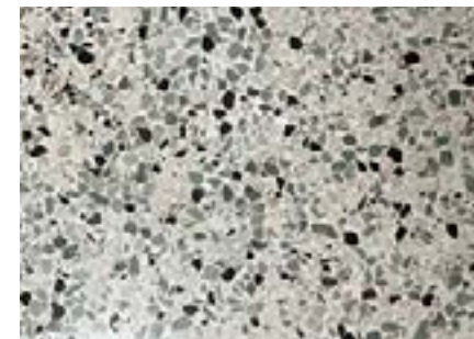
Existing Terrazzo Floor
